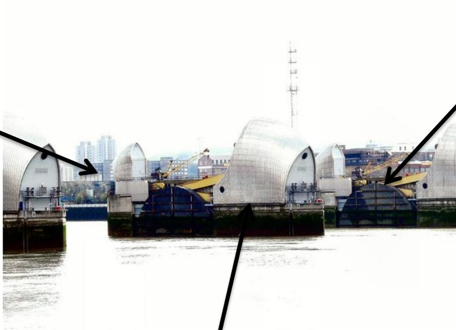
The Thames Barrier consists of 10 gates which open and close in response to tidal activity. All the gates are hollow and made of steel up to 40 millimetres (1.6 in) thick. The gates are filled with water when submerged and empty as they emerge from the river.
